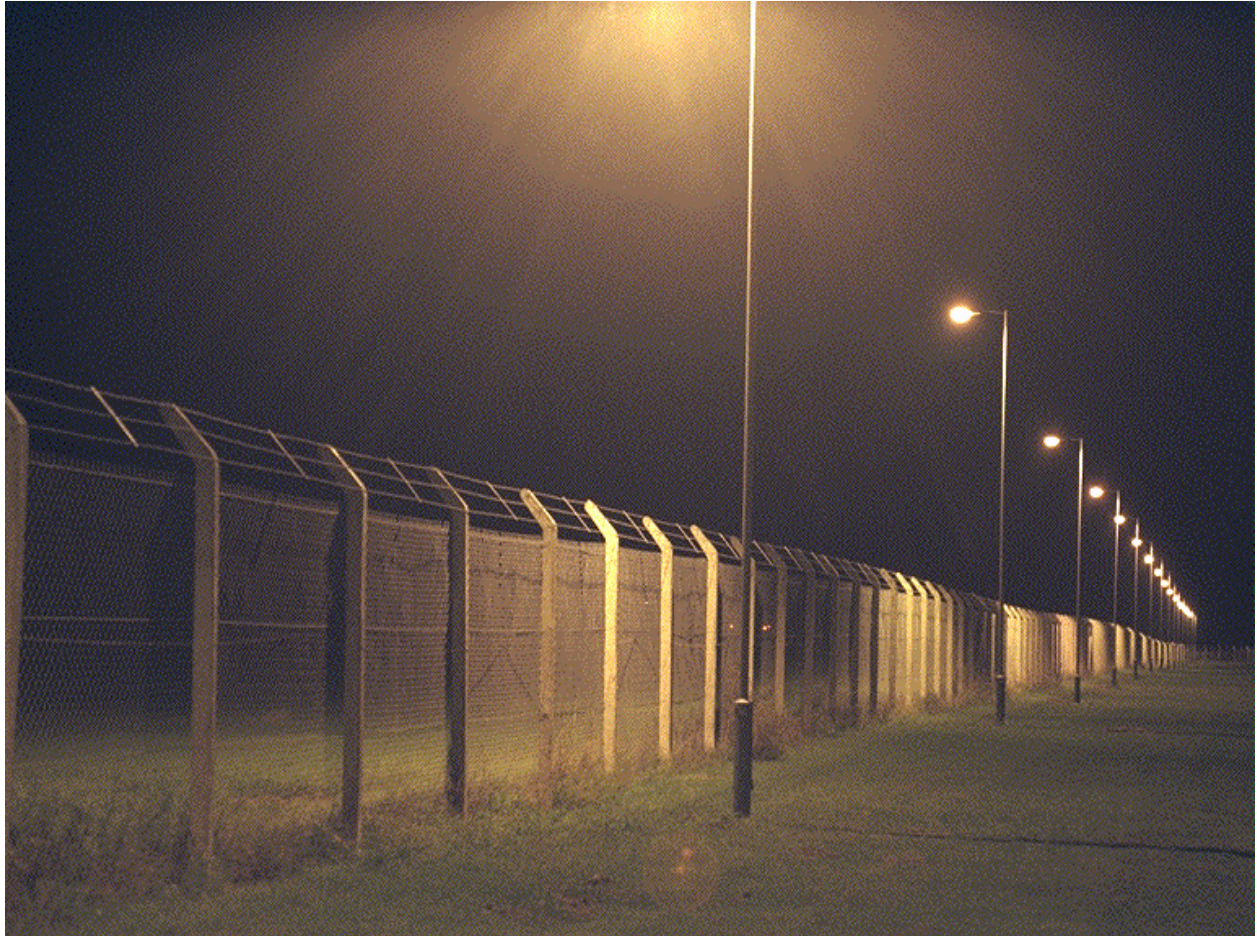
Example of perimeter lighting.
